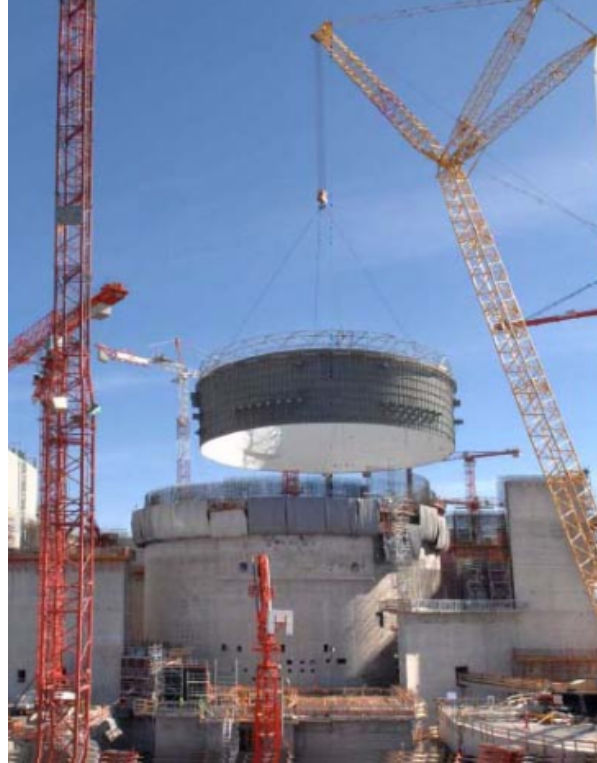
Figure 3.9 VHLC installing the containment liner for Olkiluoto 3 in Finland [36]
