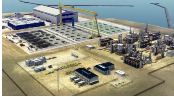
Fig. 8.3. Hydrogen Gigafactory with Factory in Back, Reactor Field in the Middle and Hydrogen Plant in the Front (Courtesy of LucidCatalyst [2020])
