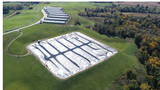
Covered Swine Manure Lagoon AD near Albany, MO
