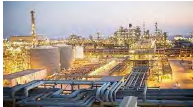
Shell Natural Gas-to-Liquids Fischer-Tropsch Plant, Qatar: 260,000 Barrels/day
