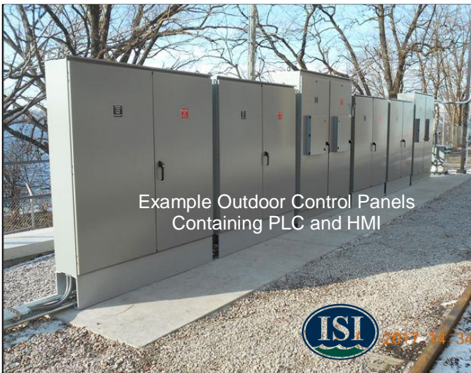
Figure 2. Intake Screens, Inc. Typical Programmable Logic Controller (PLC), Control Panels and Touch Screen Human Machine Interface (HMI)
